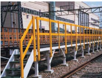
Steg einer Waschanlage Deck of a car washing area
