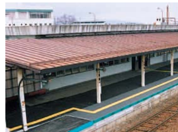
Zugangsplattform Platform raising work
