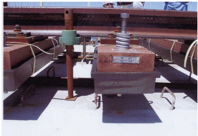
Fig. 12: Detail of rubber embedded FFU synthetic wood at slab track switch, Japan
