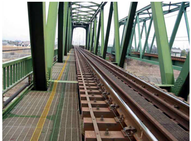
Fig. 14: FFU synthetic wood bridge sleepers on open steel structure, Japan
