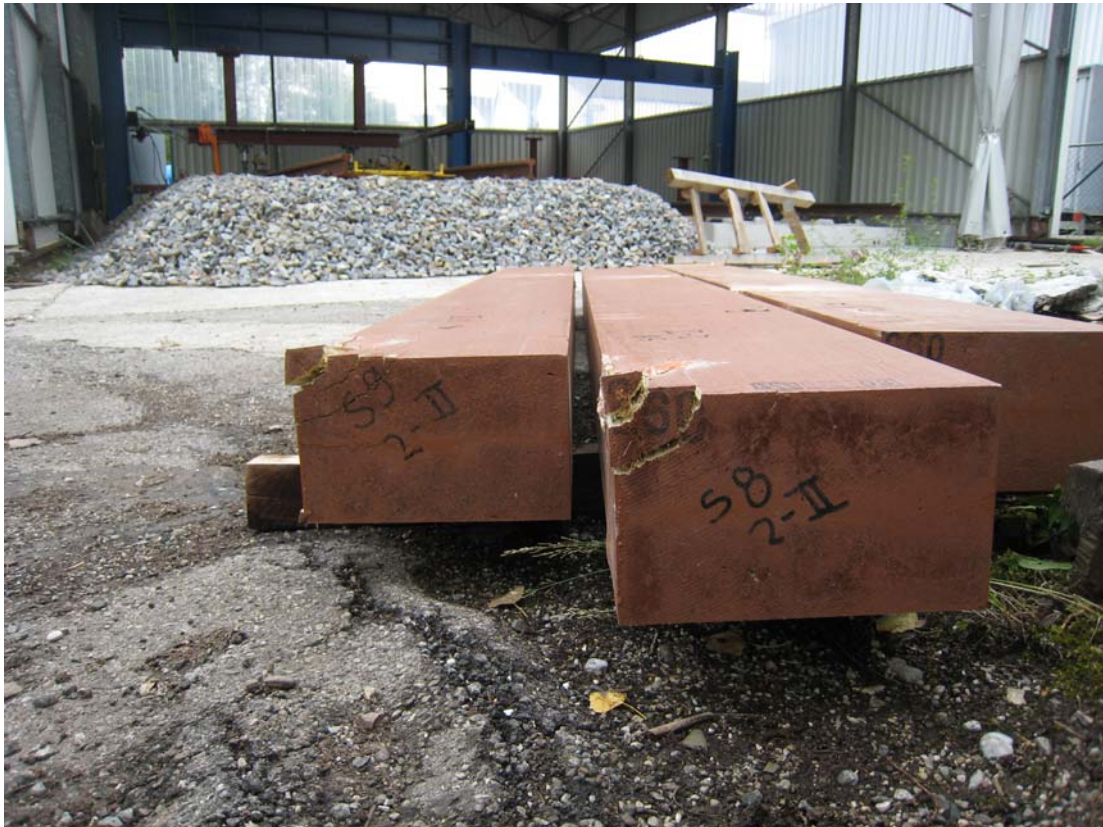
The synthetic sleepers do not show any warping after the derailment test.
